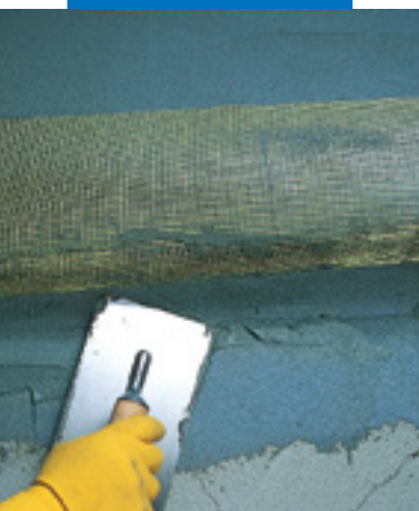
Waterproofing with Mapelastik reinforced with Fibreglass mesh
